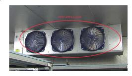
flow and cause the coil to ice up. In addition, stacking product too closely to the door thermometer can give false readings.
